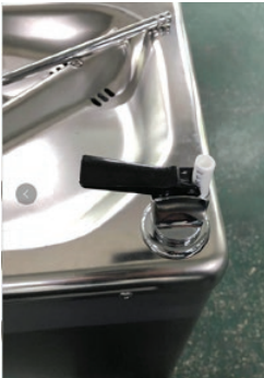
Glass filler installation
